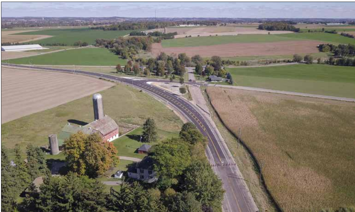
The construction project to improve safety in the Punkeydoodles Corners area is close to completion. Oxford County expects it to be open to motorists within two weeks. Photo by Dave Snooks
