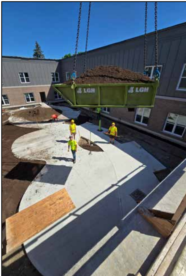
peopleCare's new Tavistock home recently had its outdoor courtyard filled with topsoil. The dirt was brought in via a large steel bucket hooked up to a crane. Contributed photo
